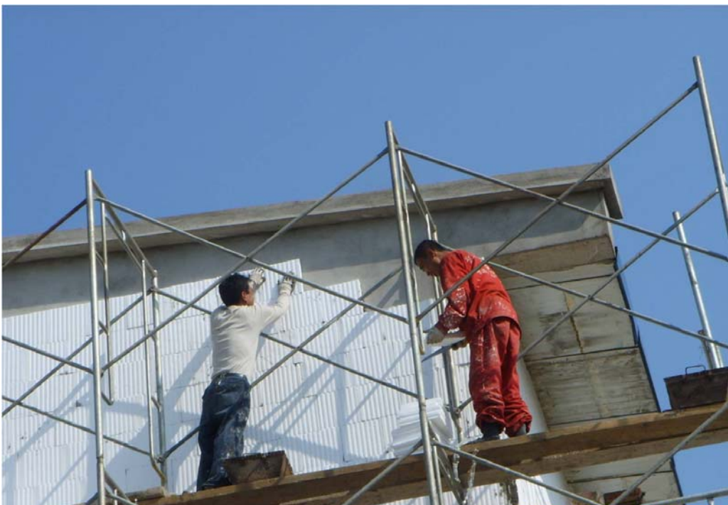
Picture 5: EPS insulated wall
